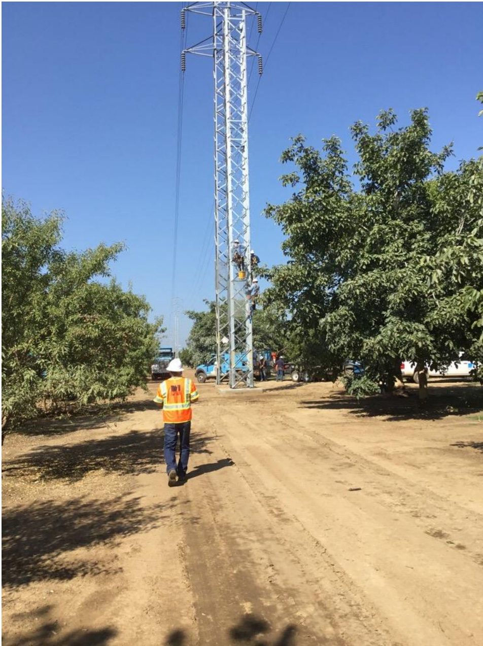
Photo 2: Tower installation Bogue Sub-Line Segment Pole 4/35.
