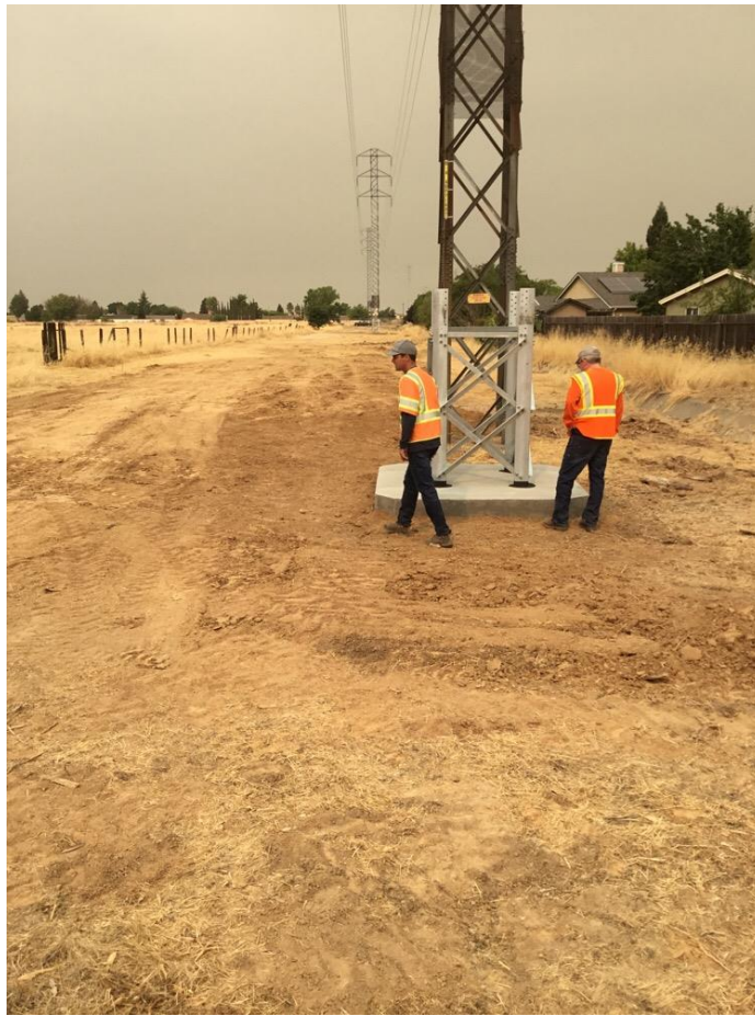
Photo 1: Completed foundation at Bogue Sub-Line Segment Pole 0/4.
